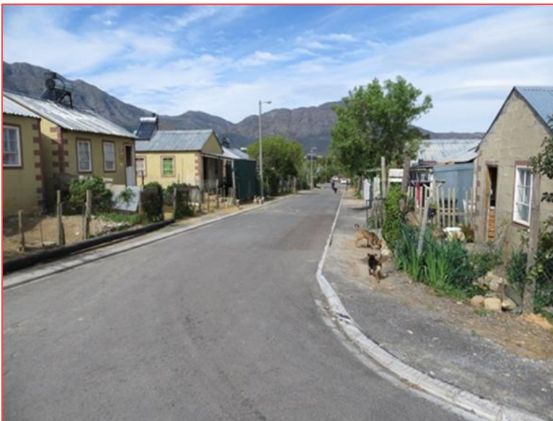
Figure 6-158: Example of completed road in residential areas
